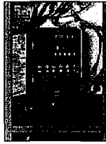
7-Day Timer turns heater and skimmer on and off at pre-set times
